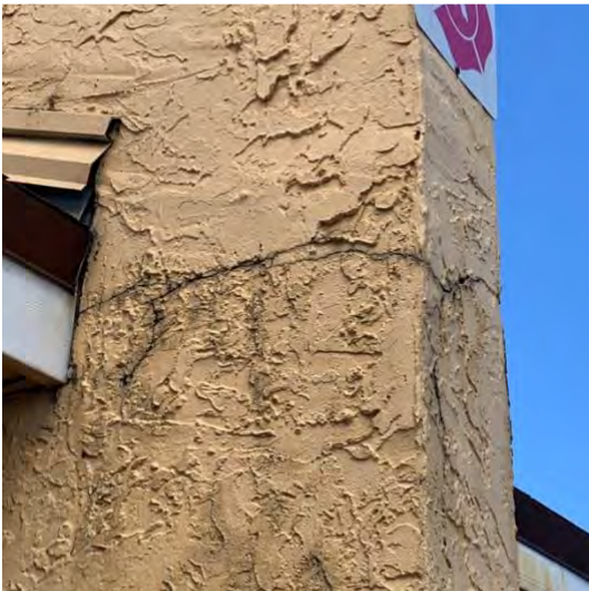
Cracks in Stucco to Patched
