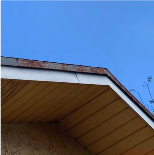
Bare Metal Flashing to be Spot Primed
